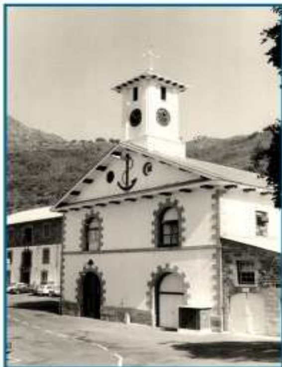
The Mast House and Sail loft (photographed c.1960) is seen to the left. One of the first Admiralty buildings designed and built by the Royal Engineer in 1815 and who saw no need to take their design inspirations from the past building norms of Simon's Town. Notice rather the employment of new Regency design elements of a shallow pitched roof and rusticated quoining on the corners and around the apertures of the building as well as the curved/arched windows and doors. Some of these innovative features can also be seen on the historic storehouse (behind, to the left) which the Engineers added a floor and other alterations and additions to during this early period of British command in Simon's Town.
