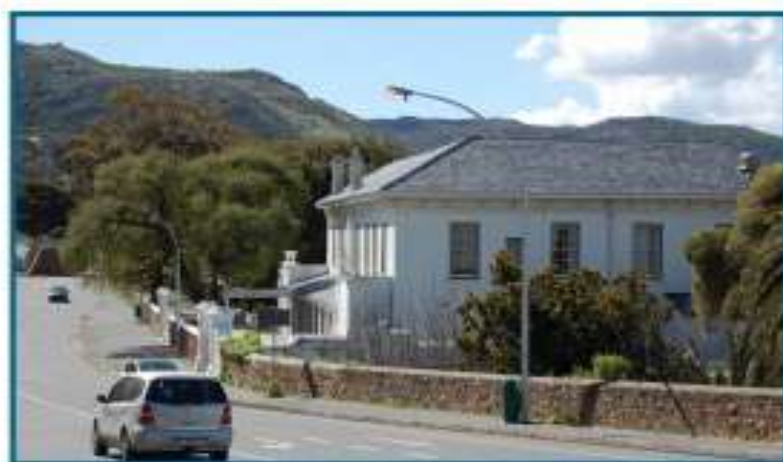
Admiralty House seen to the left carrying a flat Georgian parapet roof as painted by Christopher Webb Smith c.1838 (courtesy of the Library of Parliament) and above as seen today with its pitched roof, of trussed timber frame and tiles of blue Welsh slate added in 1875.
