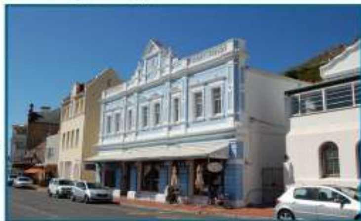
Today's Runciman Building
