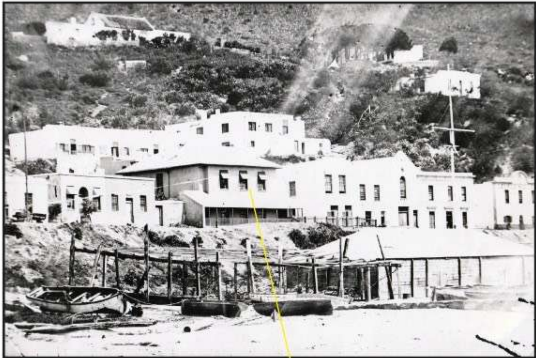
A photograph of the area in question taken from Cole Point (c. 1880). Notice the building in the centre of this picture which was the original Anglican rectory. Today (minus its pitched roof and with the addition of an enclosed balcony) this building serves as the much altered local landmark - Kalidas clothing shop. (Courtesy of Simon's Town Museum)
